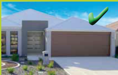
Correct: Rendered walls with rendered posts
