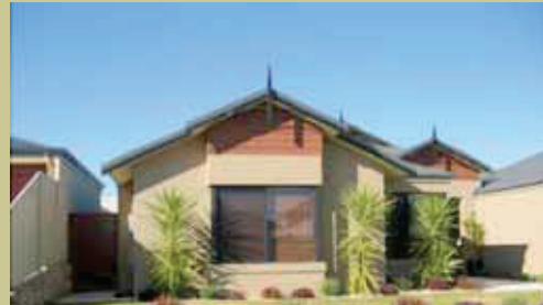
Gable with feature timber panelling
