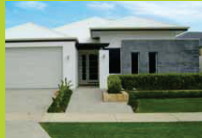
Contrasting wall materials
