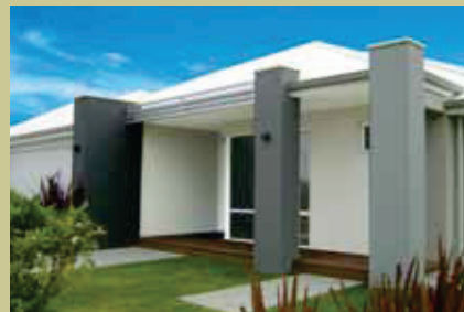
Contrasting painted walls and feature bollards
