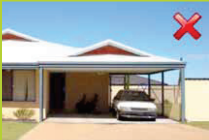
Incorrect: Brick walls with metal posts
