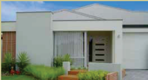
Contrasting feature walls and modern verandah
